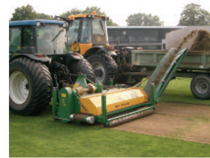
1. Planing off the surface to establish a primary level
