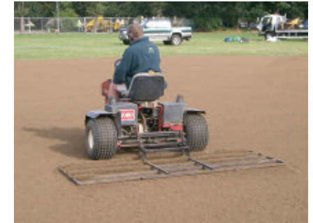
4. Grading to level
